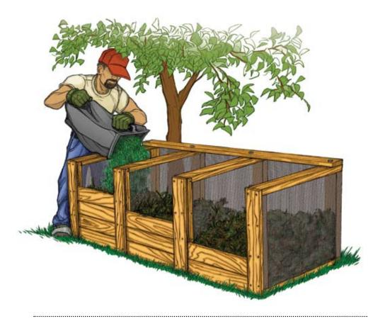
**Step 6:** Cut one 9' piece from the 10' construction-grade 2x4. Attach this 9' board to the back side of the top of the composter using the process in Step 5. With a carpenter's square, or by measuring between opposing corners, make sure the bin is square. Tighten all the carriage bolts securely.
